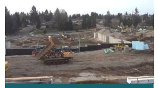
Our expansion is moving right along. All of the foundation walls of our new Health Care / Memory Care building have been poured, and many loads of gravel and soil are being brought in to backfill the foundation walls and to begin leveling the North end of the building's footprint.
