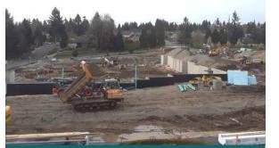
Our expansion is moving right along. All of the foundation walls of our new Health Care / Memory Care building have been poured, and many loads of gravel and soil are being brought in to backfill the foundation walls and to begin leveling the North end of the building's footprint.
