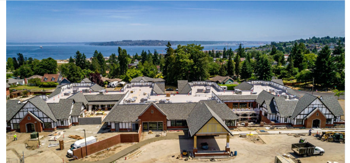
New Franke Tobey Jones Care Center with Skilled Nursing and Memory Care
